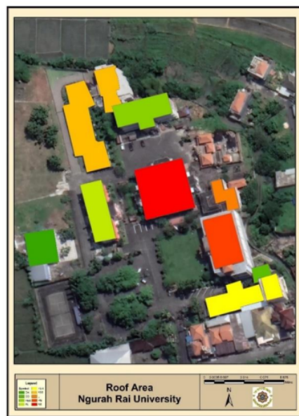
Figure 2. Analysis of roof area in study site building
